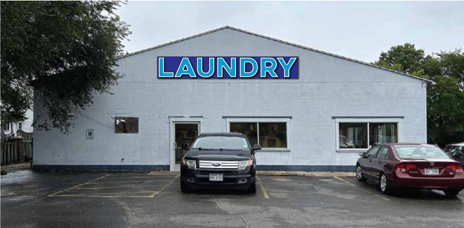
New letters installed
