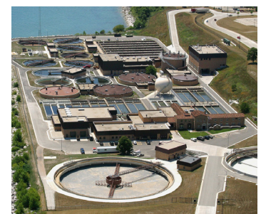
WWTF Upgrades City of Racine, WI $2M in Principal Forgiveness
