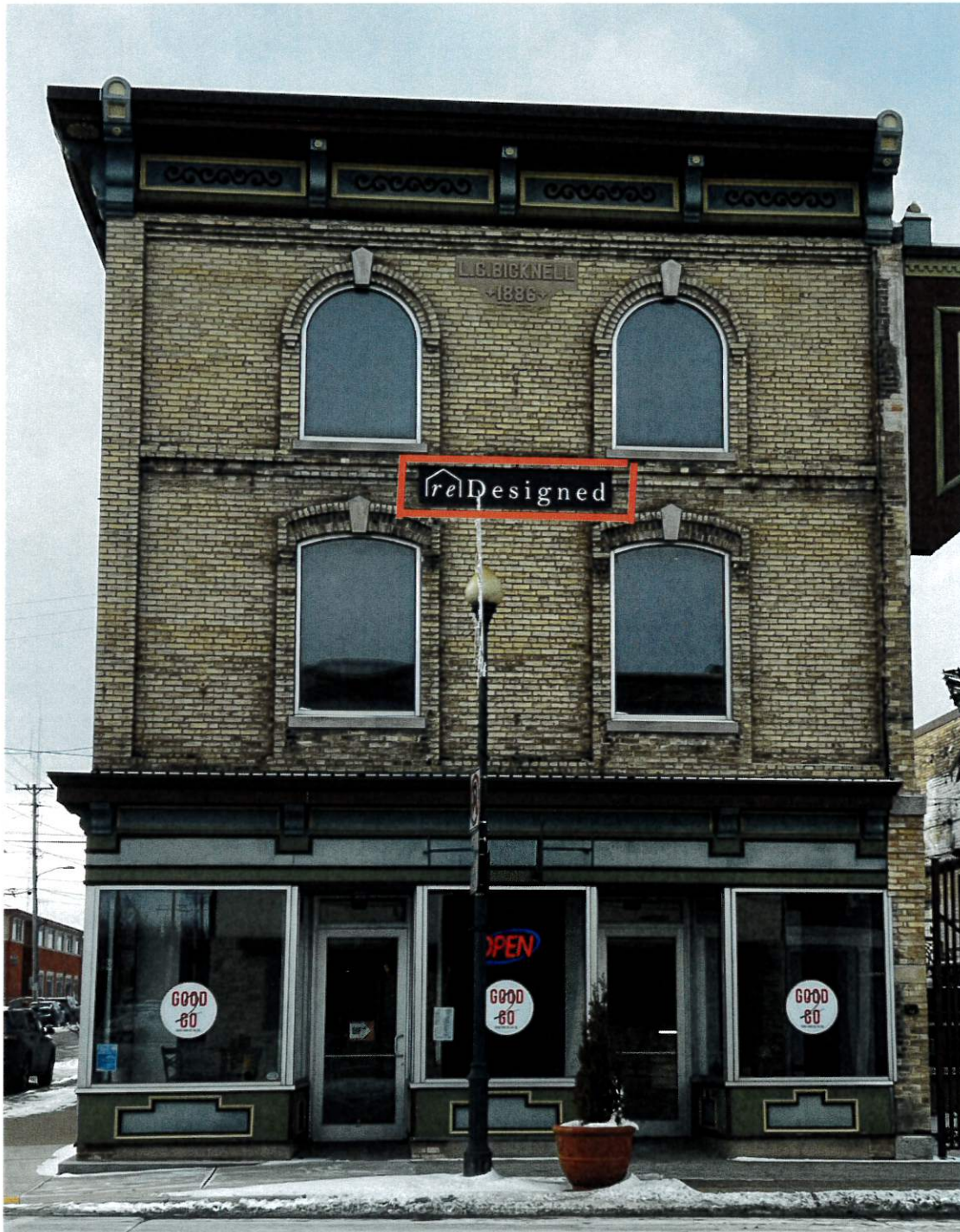
96 S. Main Street, Unit C front of building - replace current sign
