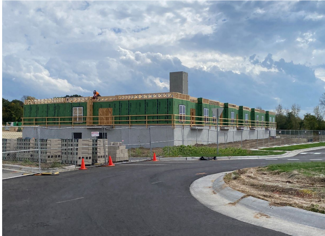
The new Ridge View Lofts building is seen being constructed in October.
