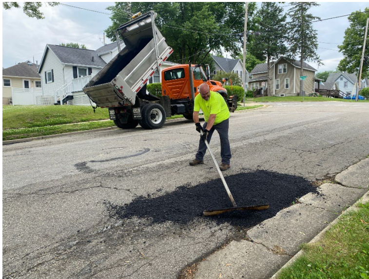
THE DEPARTMENT OF PUBLIC WORKS COMPETES PATCHING WORK ON N. FOURTH ST.
