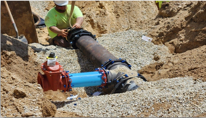
The City's contractor is seen installing a watermain.
