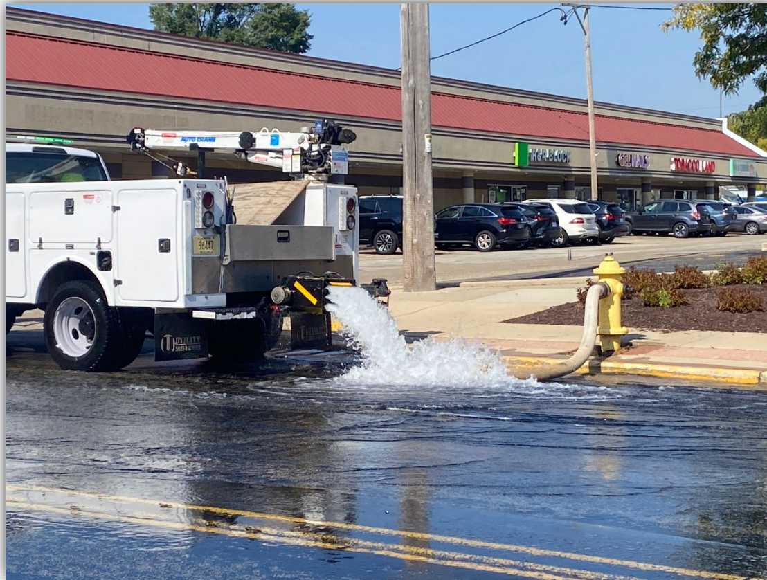
Hydrant flushing is seen this fall on Sherman Ave. W.
