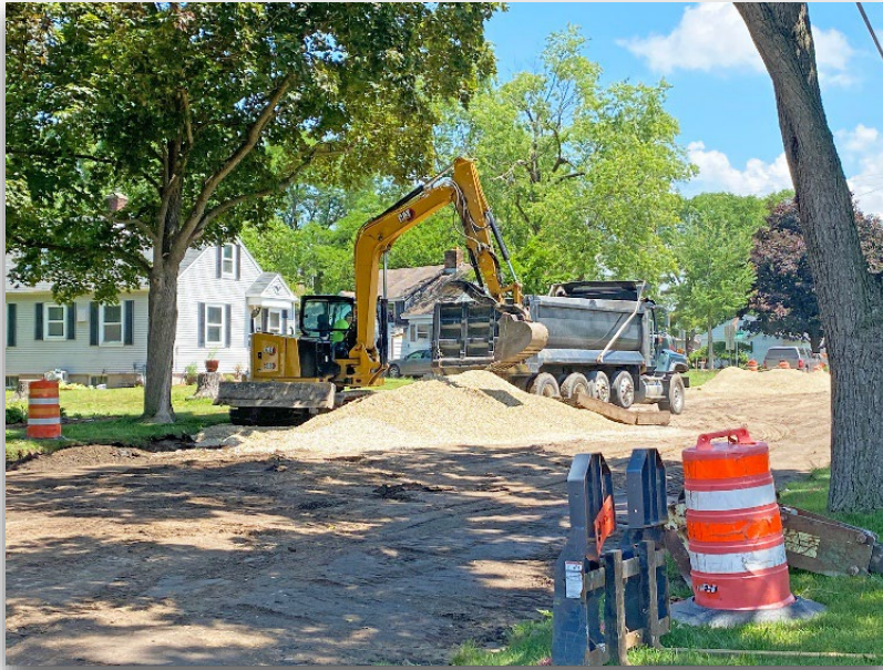
Watermain repair work is seen on the north side of the city this summer.
