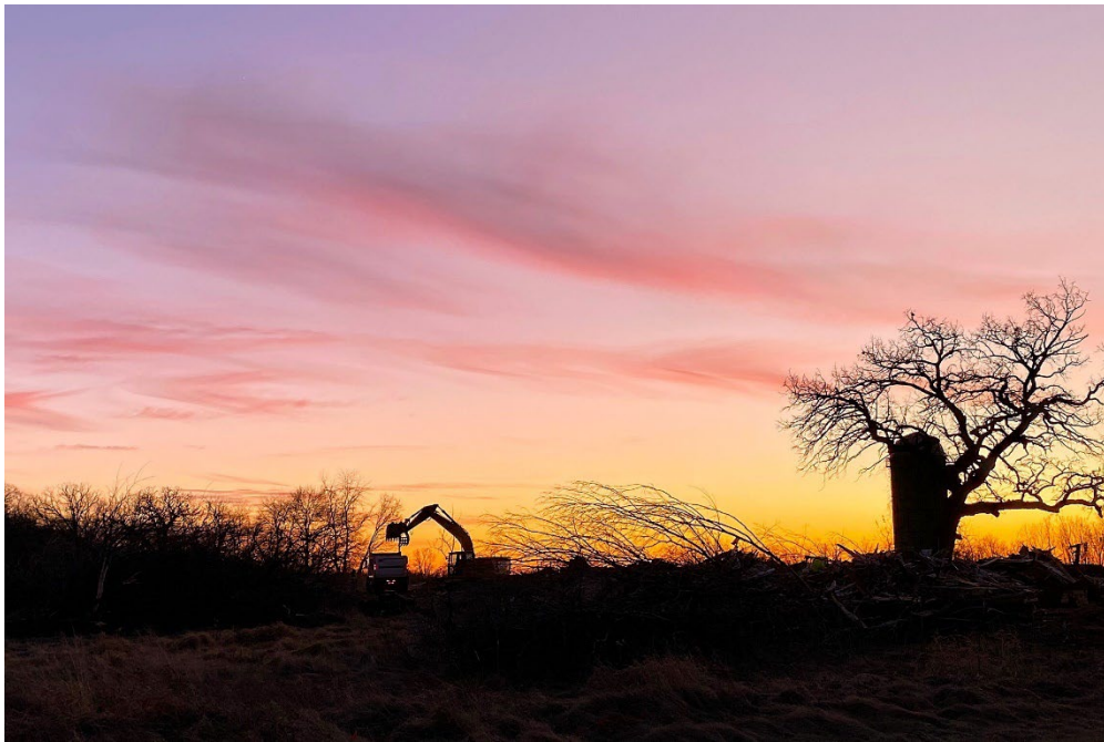
The sun is seen setting as crews work in the background clearing the Ridgeview Estates subdivision last December.
