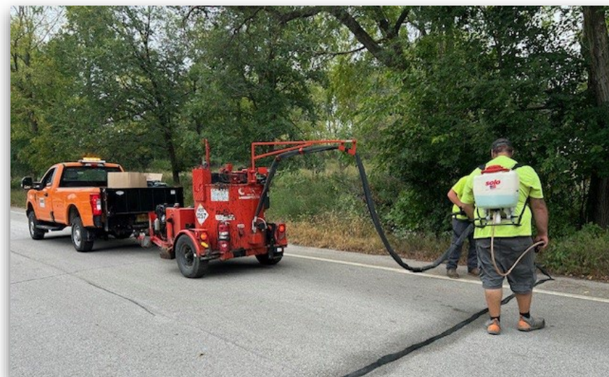
Above, members of the Department of Public Works Operations do crack filling. Below, members of the Department of Public Works Operations are seen working on an asphalt roadway repair on Janesville Ave.
