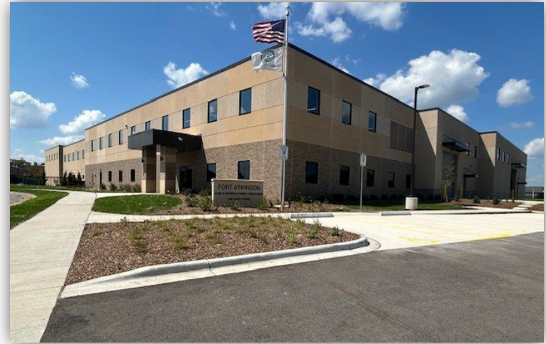
The department of Public Works and Parks Operations is seen after completion this summer.
