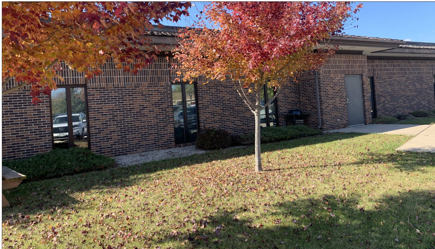
16 A4 EXTERIOR PHOTO (EXISTING NORTHEAST FACADE) SCALE: N.T.S. 2020/DRAWINGS.DWG DATE:
