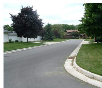
Annual Road Reconstruction & Rehabilitation Program since 2007
