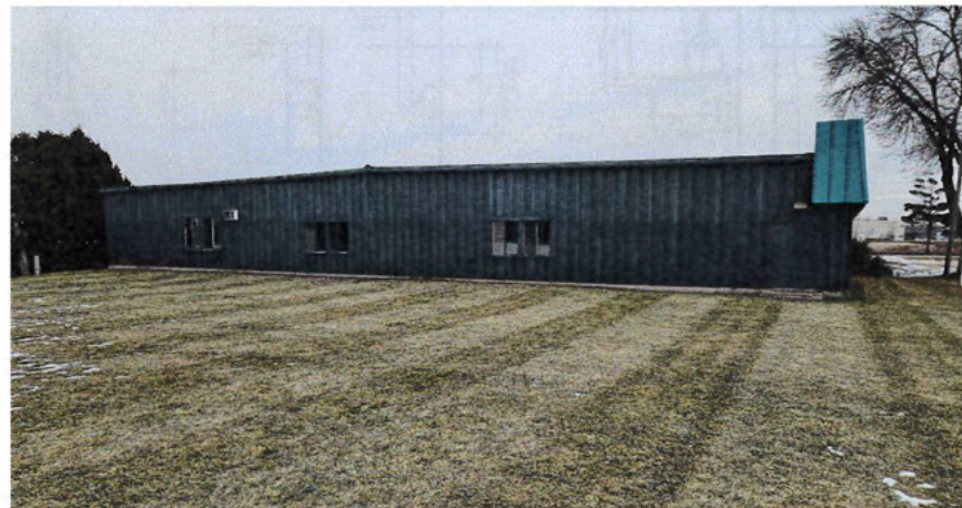
1.0 A4 EXTERIOR PHOTO - SOUTHEAST FACADE SCALE: N.T.S. 2020DRAWINGS.DWG DATE:
