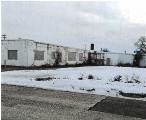
1.0 A4 EXTERIOR PHOTO - SOUTHWEST FACADE SCALE: N.T.S. 2020DRAWINGS.DWG DATE:
