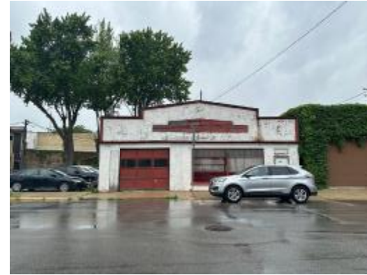
EXISTING SITE IMAGES SCALE: N.T.S. 2022/PREMIER BANK PARKING/FBP-DRAWINGS.DWG DATE: AUGUST 12, 2022
