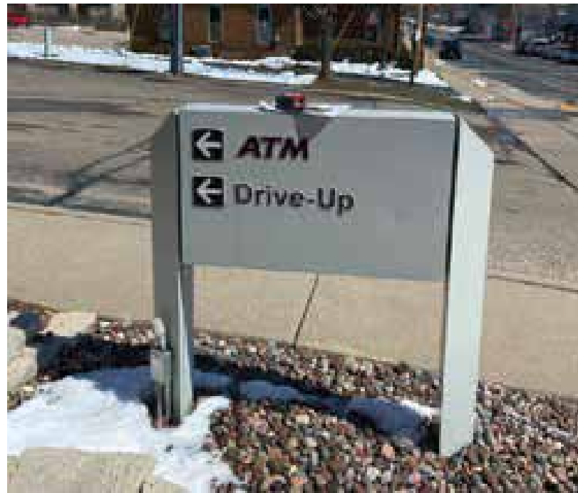
remove & replace existing sign (existing side A)
