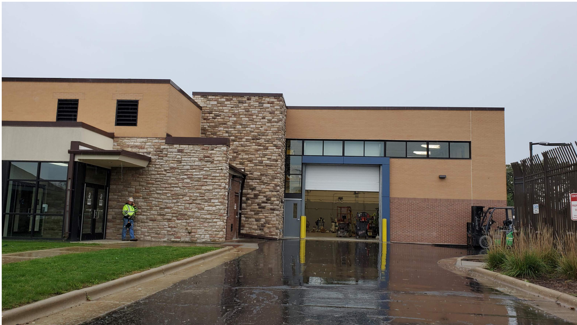
IMAGE 1 EXISTING BUILDING - NORTH FACADE, METAL FABRICATION LAB ENTRY
